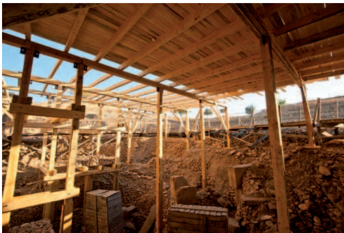
The wooden shelter during construction (Photo: NB).
