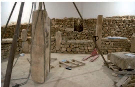
The re-construction of the Nevalı Çori “Temple” (Photo: MA).
