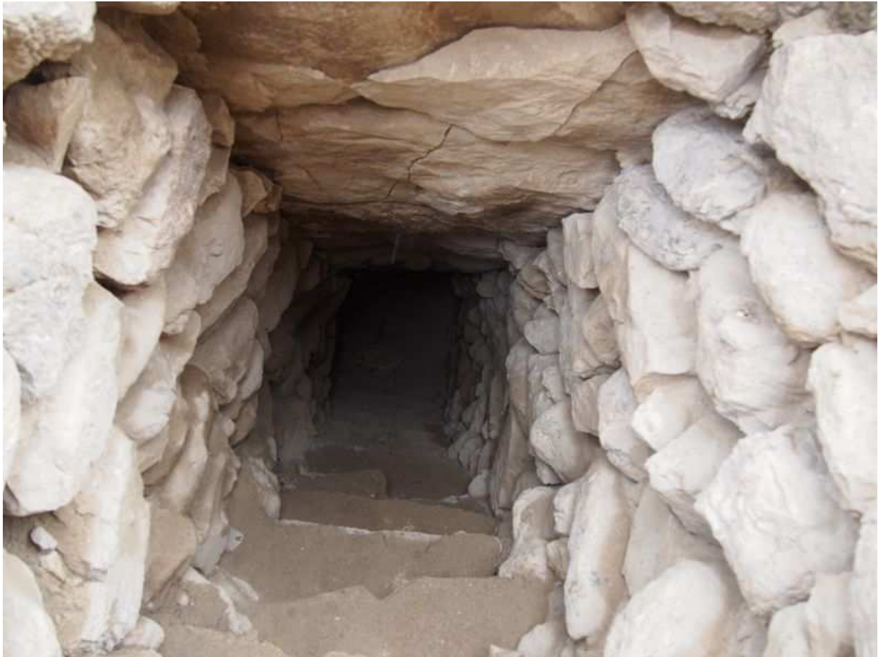
Figure 8.d. Tower of Jericho, the interior of the staircase. This modest shaft's Architecture is of great significance, as it carries far reaching implications for the Neolithic monumental Architecture of the entire Eurasia. Lintels were used for the first time in forming the roof of the shaft, a narrow passage, containing the staircase of approximate 80x80 centimeters. These are possibly the first lintels used in any human monument. However, the presence of lintels must be construed as evidence that this is a later than the 8000 -7000 BC structure (as claimed by K. Kenyon). The staircase contains 22 steps, reaching about three quarters down the tower's height. The rough masonry ashlar structure of the side walls is noted. Source of photo: ref. [2.48].
