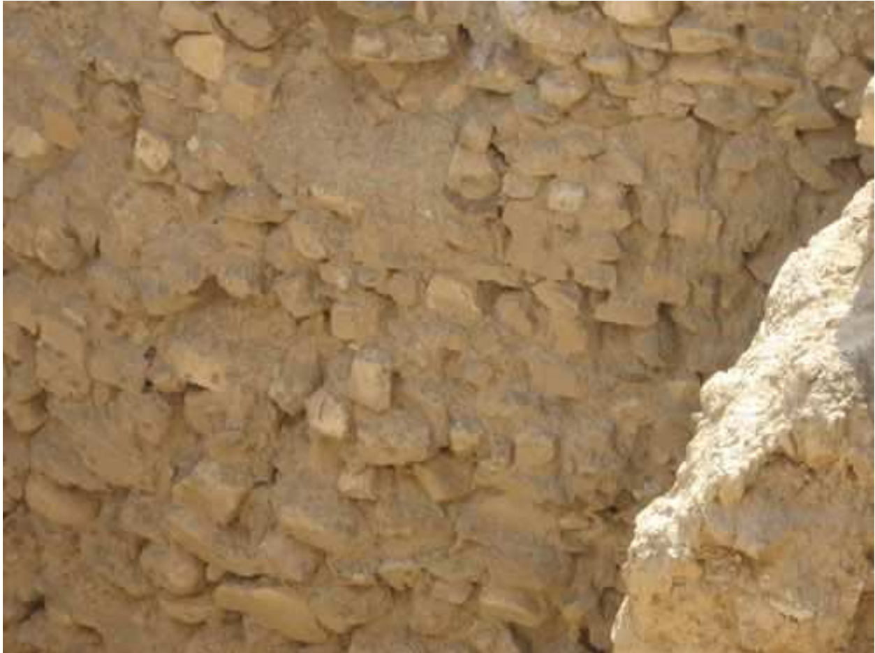
Figure 10. Tell Es-Sultan. The construction detail of the structure called the “tower of Jericho”. Masonry dry ashlar irregular blocks and small stones plus mudbrick with mud filaments was the way that the exterior surface of the monument was finished and dressed. This is in sharp contrast to the manner in which the masonry (including the two sidewalls, roof and steps) staircase (see Figure 8.d) was enclosed. Source of the photo: ref. [2.21].
