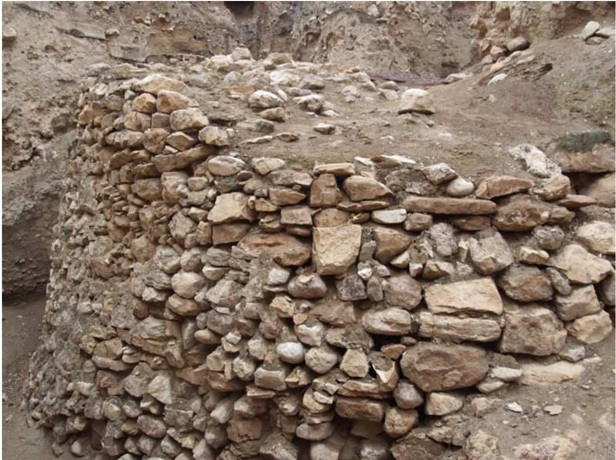
Figure 8.c. Tower of Jericho, masonry detail: different size boulders in dry ashlar, irregular leveling construction. The detail shows (at lower right) how the wall and the tower intersect, as the two bodies' surfaces interact. That higher tower and its partial "covering" of the wall implies that at this section of the wall pre-existed and the tower followed. Source of photo: ref. [2.48].
