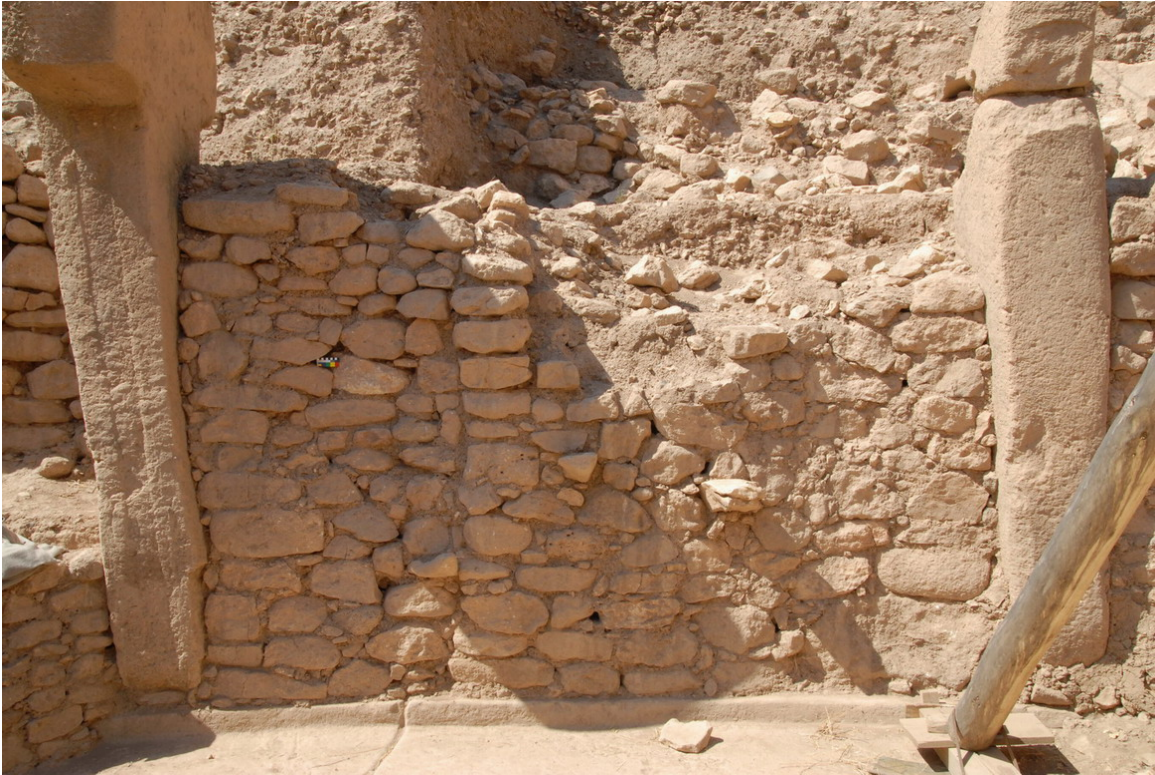
Above: Wall bay between monoliths.
