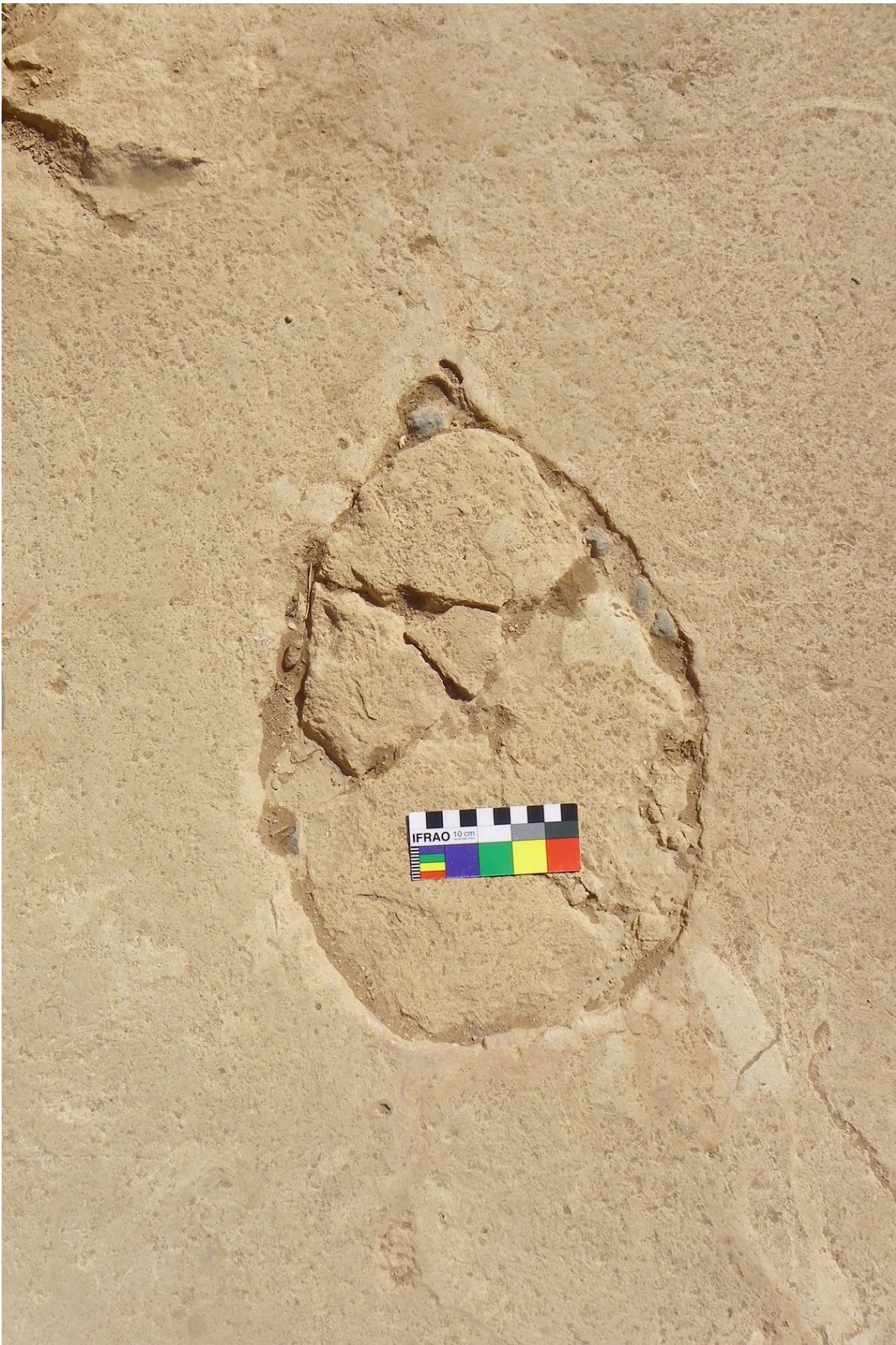
Above: A contemporary patch in stone floor with basalt wedging stones.
